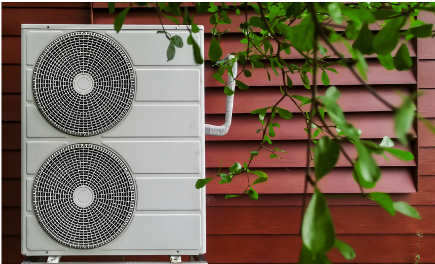
Air-to-water heat pump installed outside
